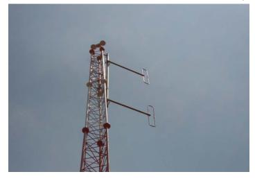
short to extremely long, compared with a wavelength. Folded antennas offers the engineer exceptional design freedom compared with other antennas. It provides independent design variables than a simple linear radiator of the same length. They are, base load impedance, top load impedance, the differential mode characteristic impedance and the common mode current transformation ratio. In practice, extremely compact folded antennas can be fabricated.
