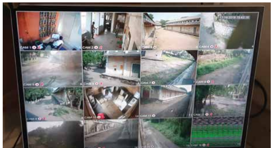
CCTV Surveillance System at warehouses of Central Warehousing Corporation
