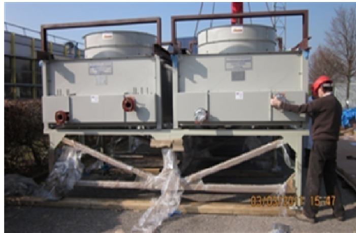
Dummy Load Heat Exchanger developed by BECIL being installed by M/s. Thomson Engineers for PDI in their works at France
